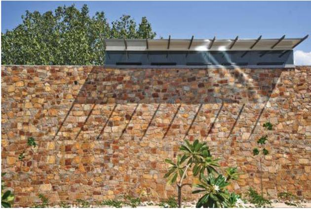
For most part, the local Rajasthani craftsmen and construction workers were employed to build in a manner rooted in the region and its landscape. Structural steel has been used as it is a long life span material, reducing dead load & thereby overall material consumption. The concrete consumption is insignificant for a building of this type and size.
