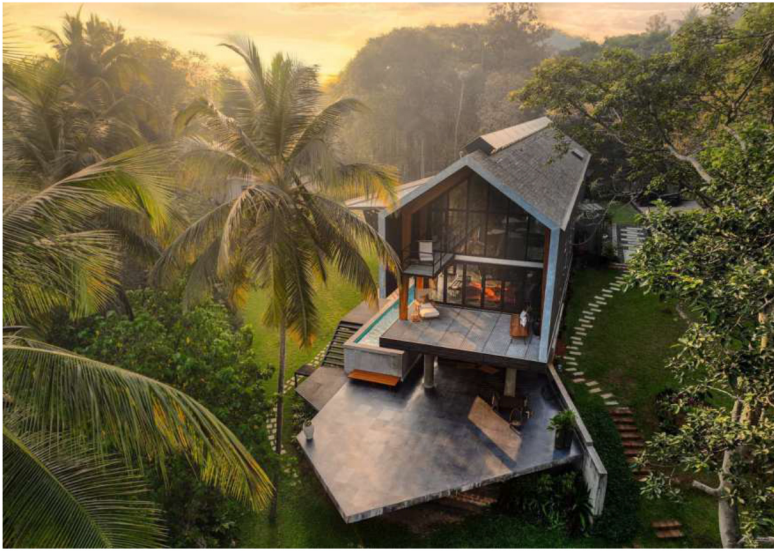
India's first mass-timber home in Vagator, Goa. STUDIO CHARULAU
